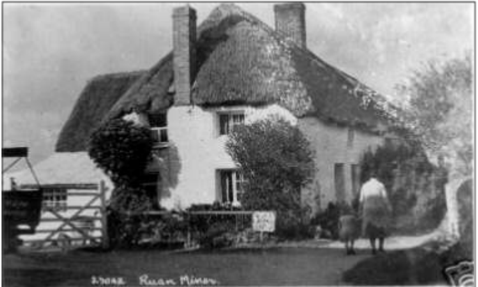
This picture is taken from the Spar end of Duck Lane, and shows the substantial Rutter Farm house, which was knocked down sometime in the 50s, as it had become derelict. Picture courtesy of Jan Morgan.
